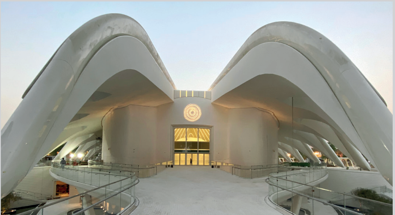
EXPO 2020 Dubai, UAE Hydraulic motion system to control the opening and closing of the roof of the UAE Pavilion
